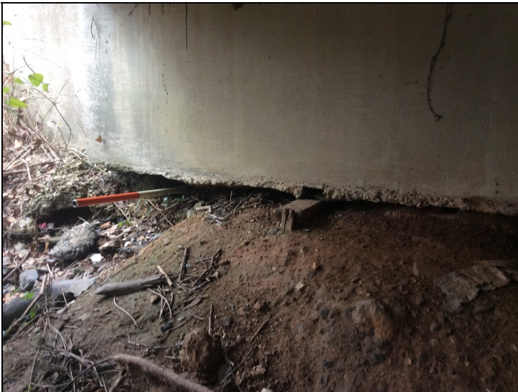
Bent 1 right side undermined due to erosion.
