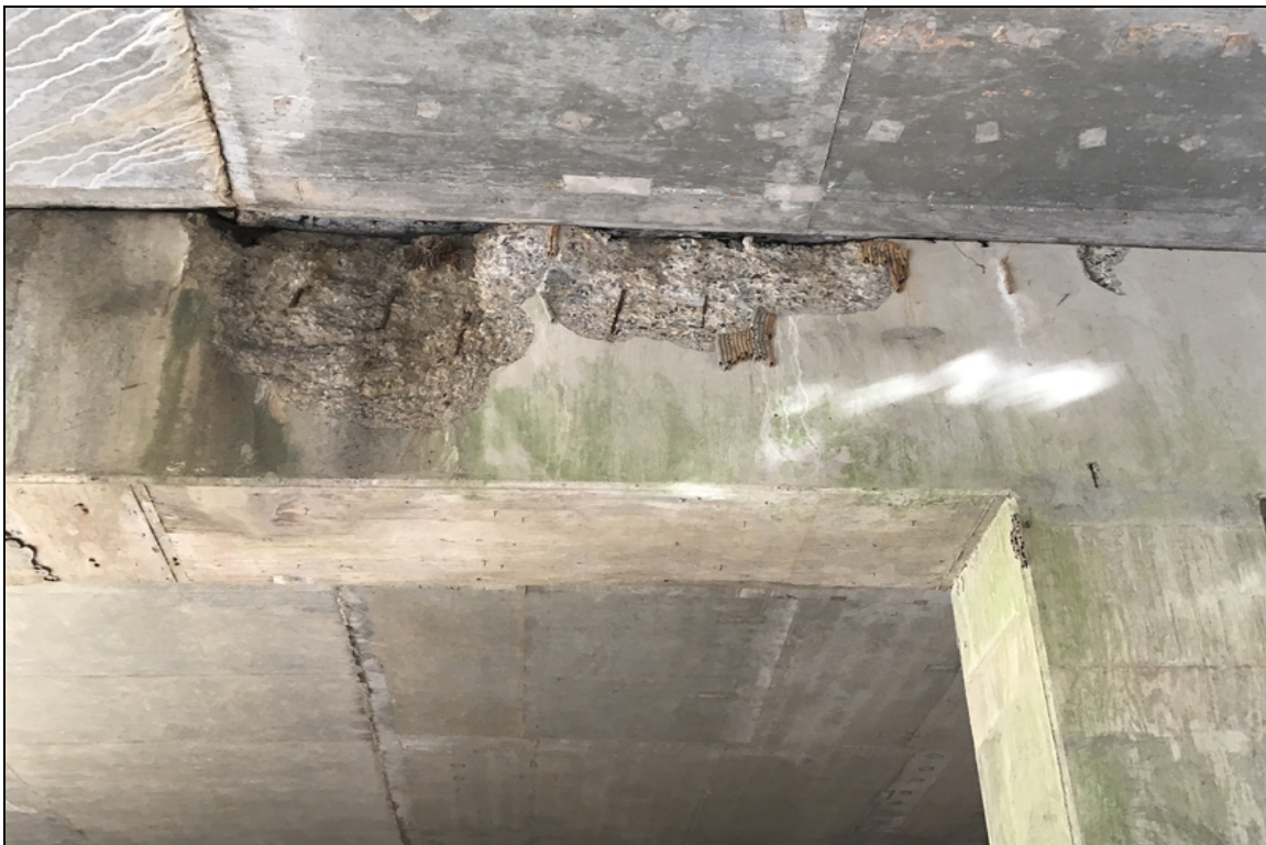
Bent 2 cap ahead has large spalls with exposed rebar.
