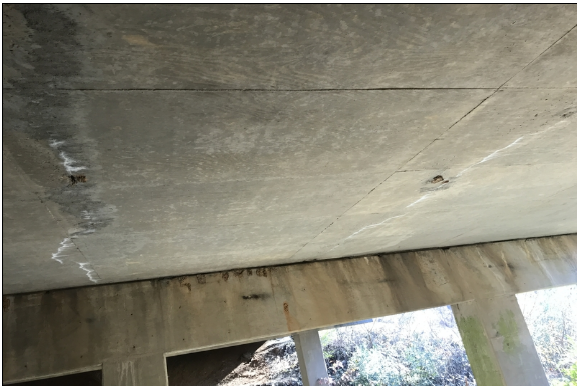
Span 1 soffit has cracks with efflorescence.
