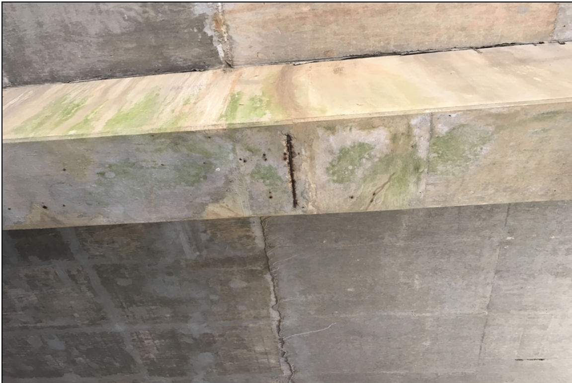
Bent 3 cap bottom between columns 2&3 has spall with exposed rebar.
