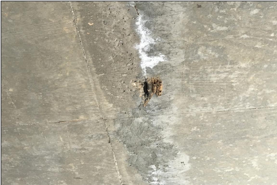
Span 1 soffit has spall with exposed rebar.
