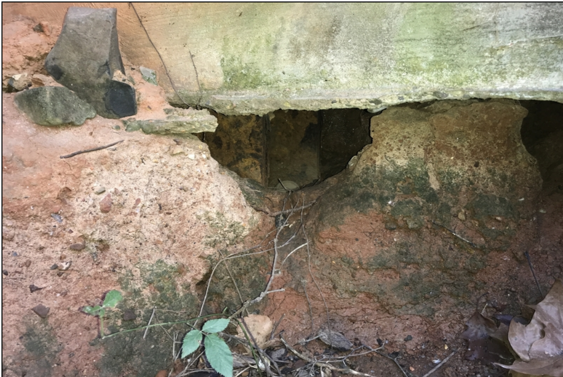
Pile exposed due to erosion on left side of bent 1 has active corrosion.
