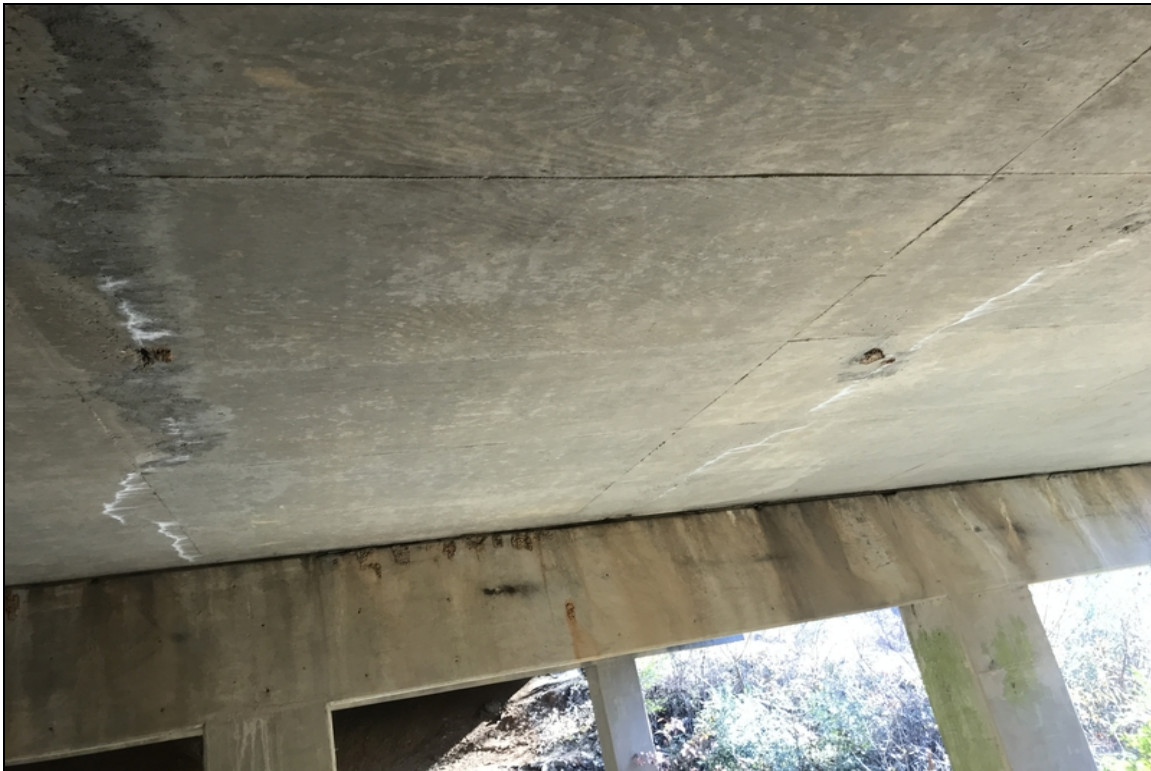
Span 1 soffit has cracks with efflorescence.
