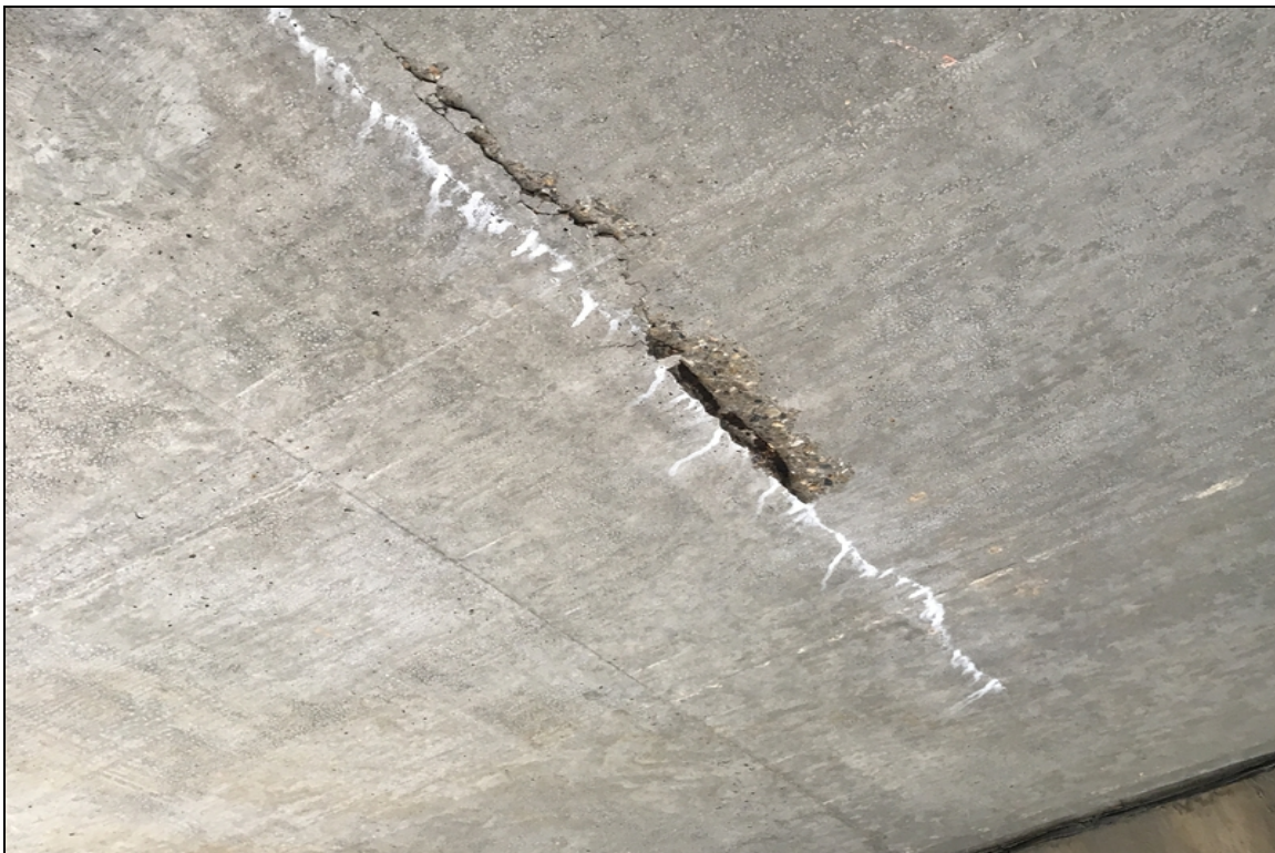
Soffit span 3 has spall with exposed rebar.
