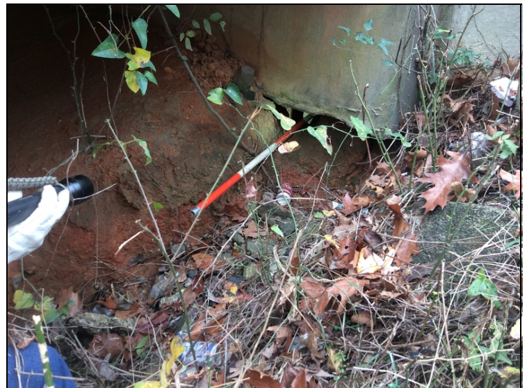
Bent 1 erosion has undermined the left end of bent.
